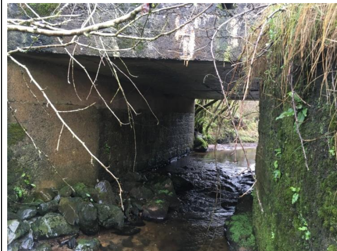
UWF Grid Connection Material haulage routes – Bridge crossing on the L2114-0 at Bealaclave
