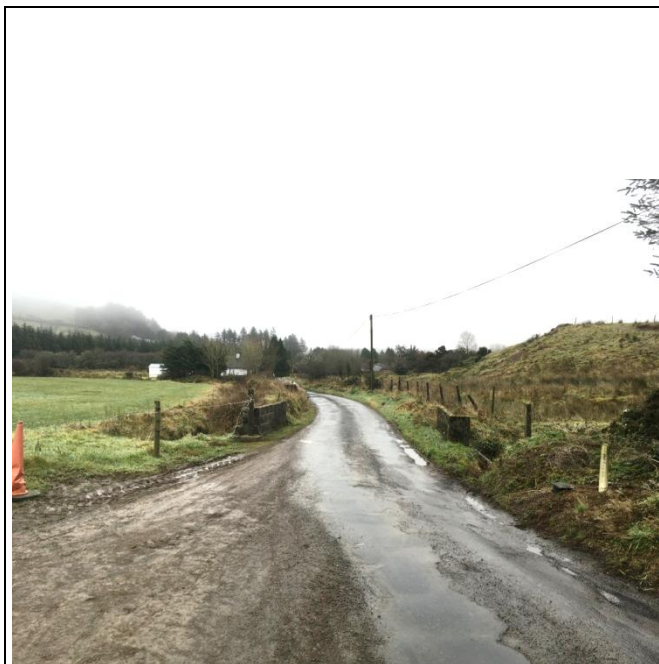
UWF Grid Connection Material haulage routes – Bridge crossing on the L6086 -0 at Laghile
