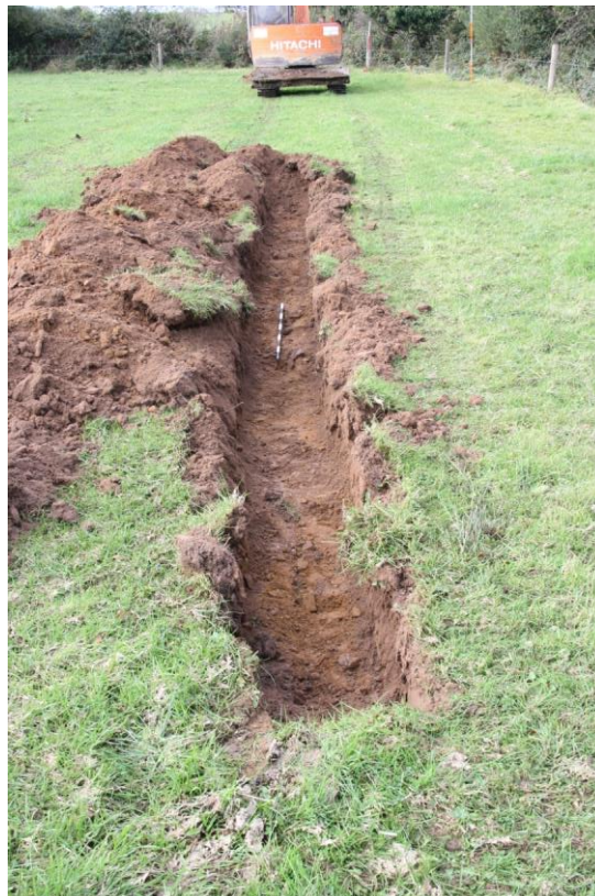
Figure 7: Test trench 2 from east
