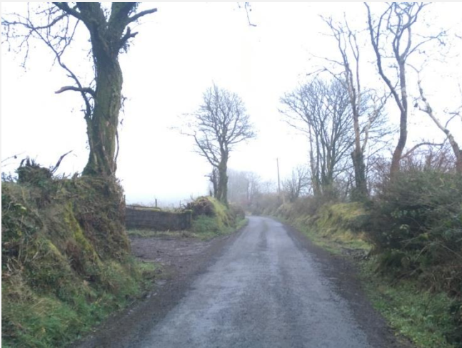
UWF Related Works Internal Windfarm Cable Public Road Crossings RW9
