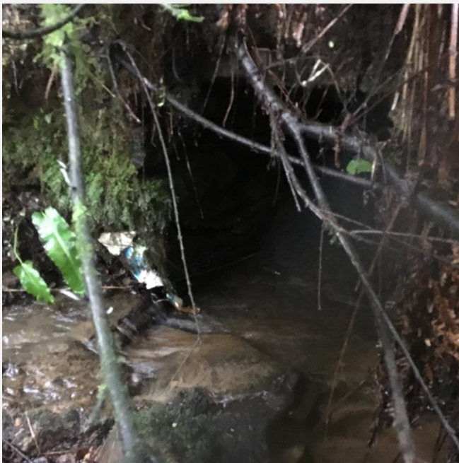
UWF Grid Connection W38
