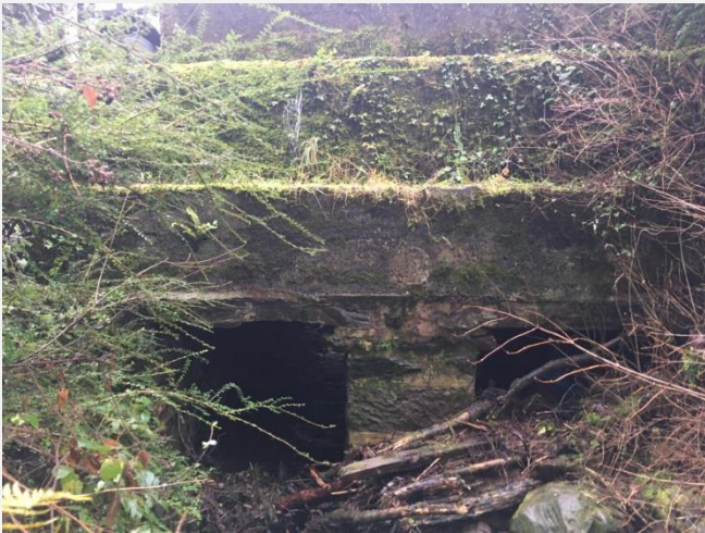
UWF Grid Connection W42
