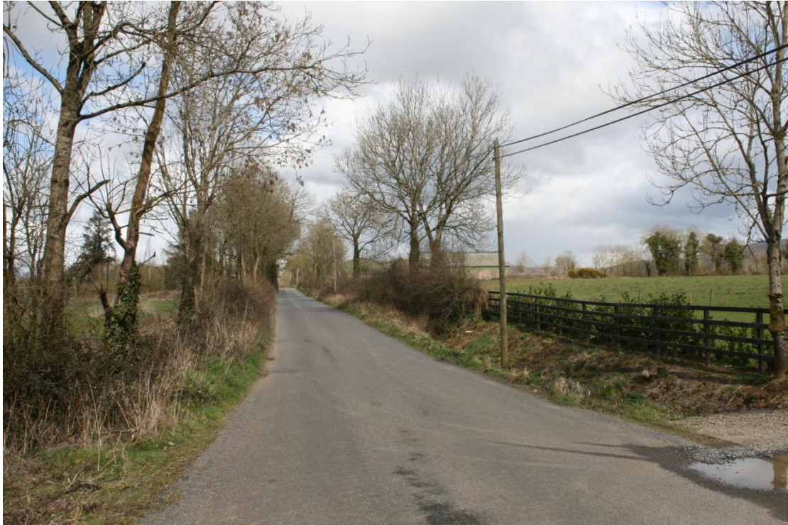
Figure 12: R002 from the south
