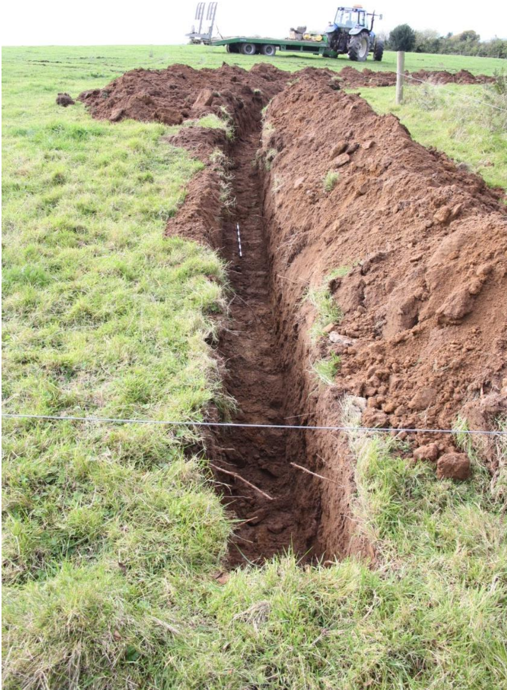
Figure 5: Test-trench 1, from east
