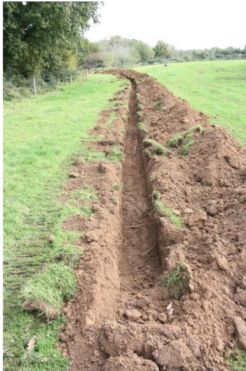
Figure 6: Test trench 1, from west
