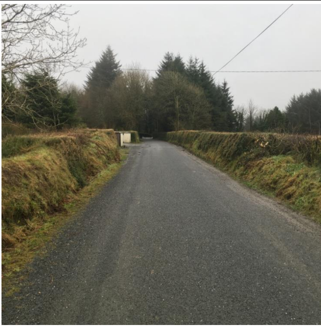
UWF Grid Connection W38
