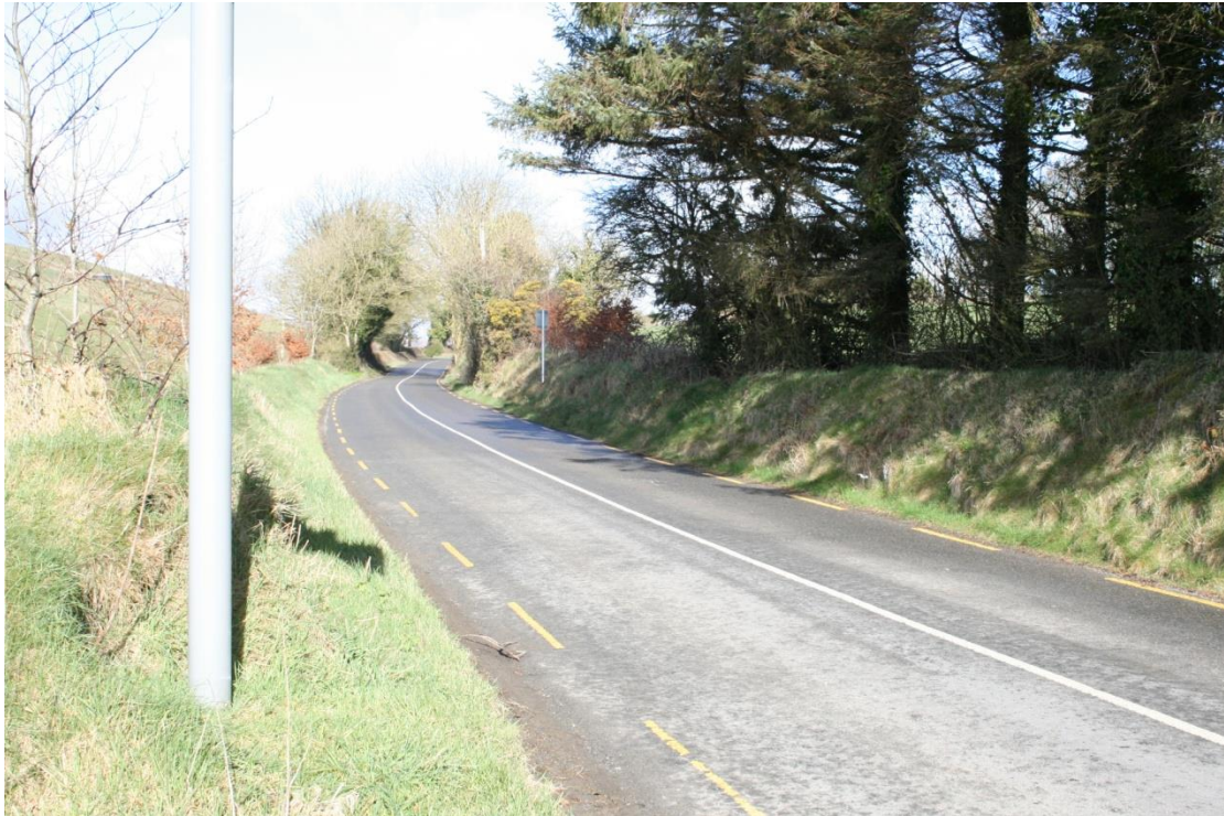
Figure 40: R012 from the south.
