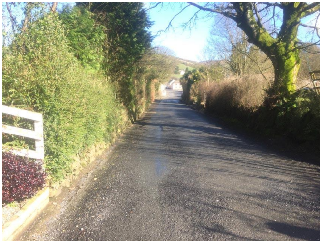
UWF Grid Connection R10
