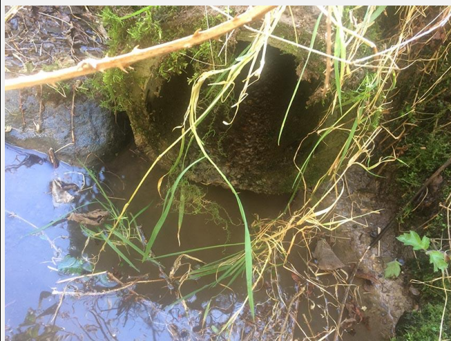
UWF Related Works Haul Route Works Bridge/Culvert Crossings WW31
