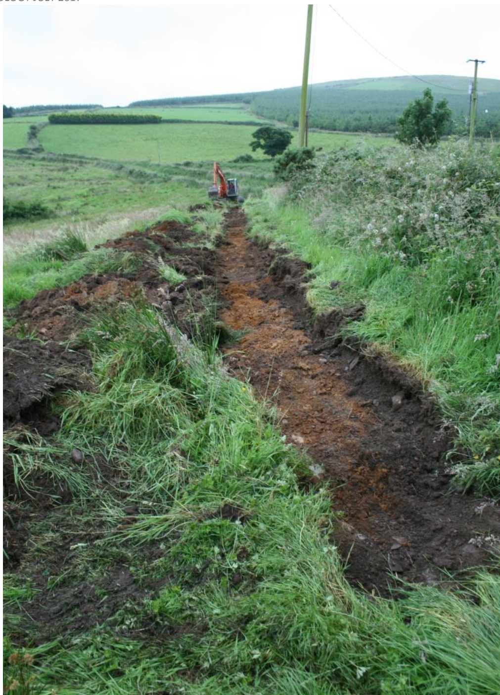
Figure 6: Trench 2 from the northeast
