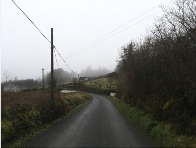
UWF Grid Connection W42
