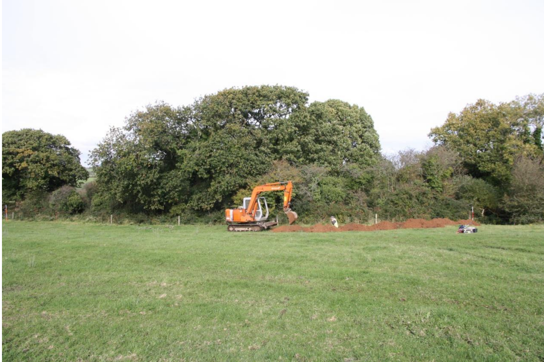
Figure 4: Test excavations underway 21st October 2016, taken from south. Ringfort TN031-067 is in the background.
