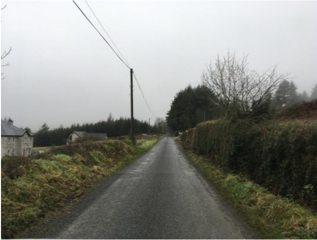
UWF Grid Connection W41
