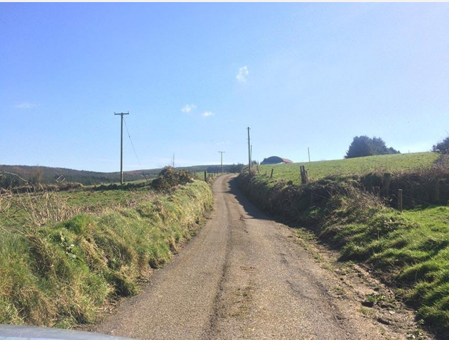
UWF Related Works Internal Windfarm Cable Public Road Crossings RW4 & RW5
