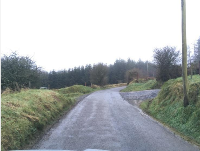
UWF Related Works Internal Windfarm Cable Public Road Crossings RW8
