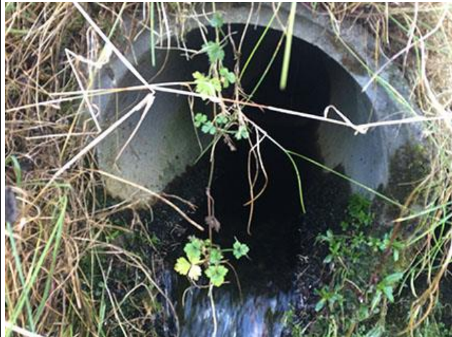
UWF Related Works Haul Route Works Bridge/Culvert Crossings WW12
