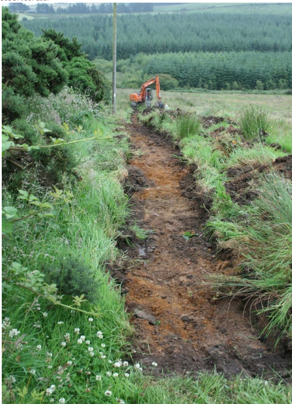
Figure 5: Trench 1 from the northeast
