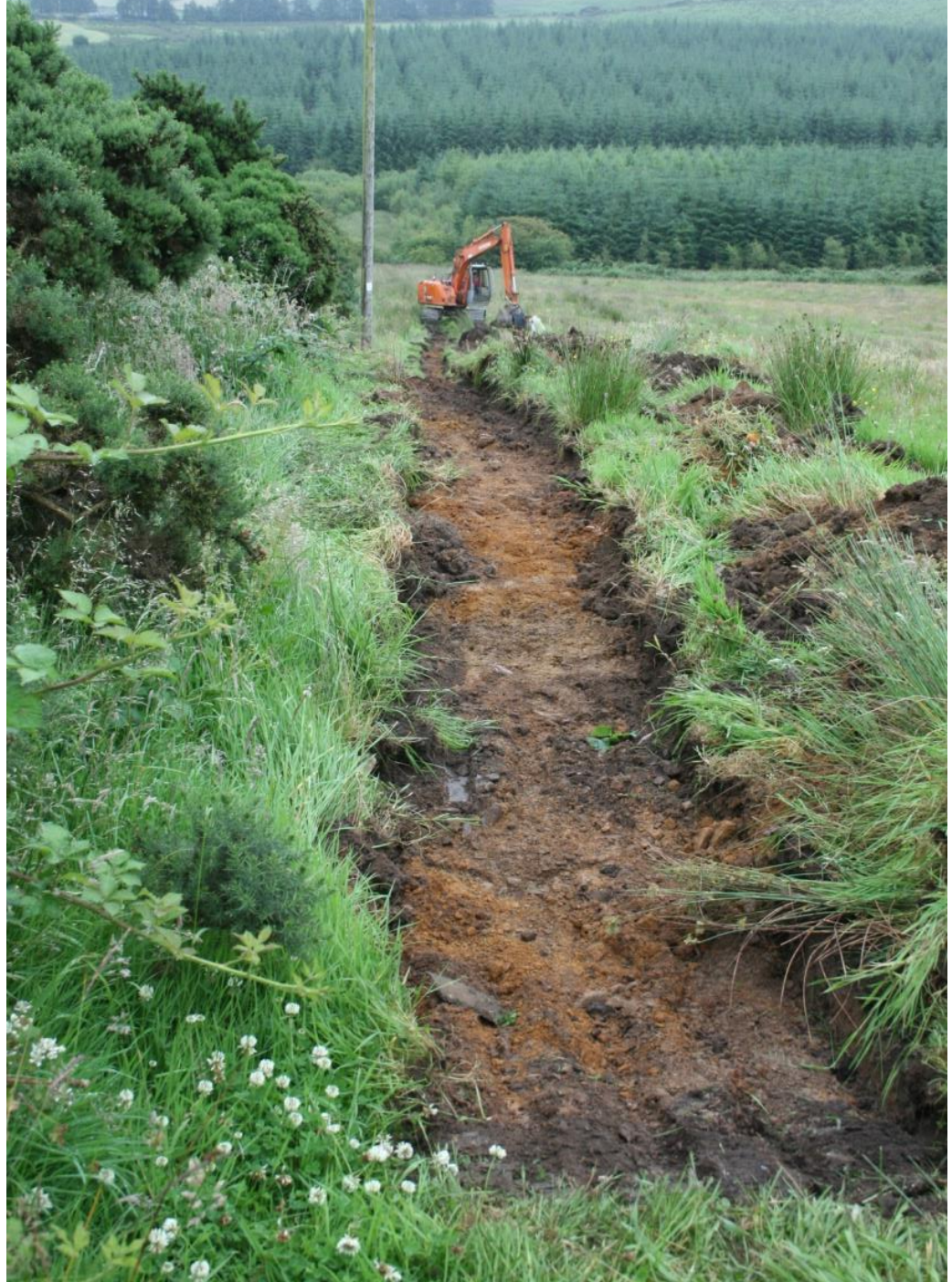
Figure 3: Test excavations underway, taken from west.
