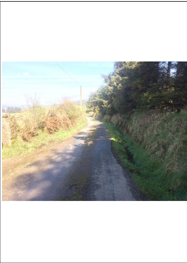
UWF Related Works Haul Route Works Bridge/Culvert Crossings WW12
