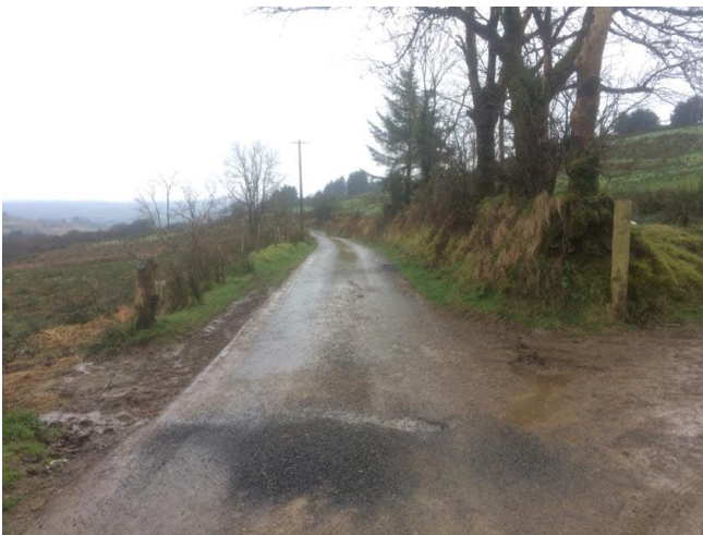
UWF Grid Connection R6
